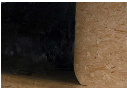
Buffer protection in the pellet depot
